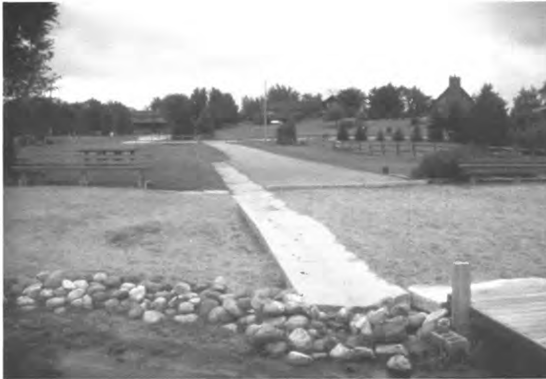
Figure 3. Constructed drain that carries surface runoff into Don Jean Bay of Mill Lake.
