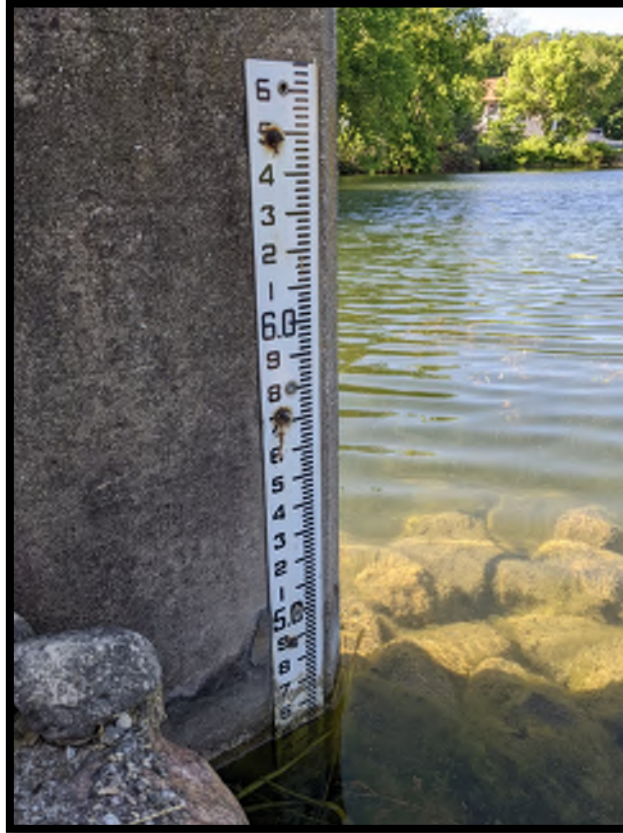
Gauge and water level on primary spillway 0021006162203.jpg
