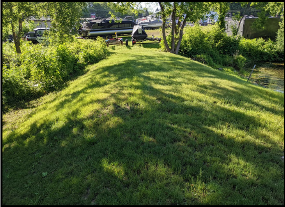
East (left) embankment looking southeast 0021006162207.jpg
