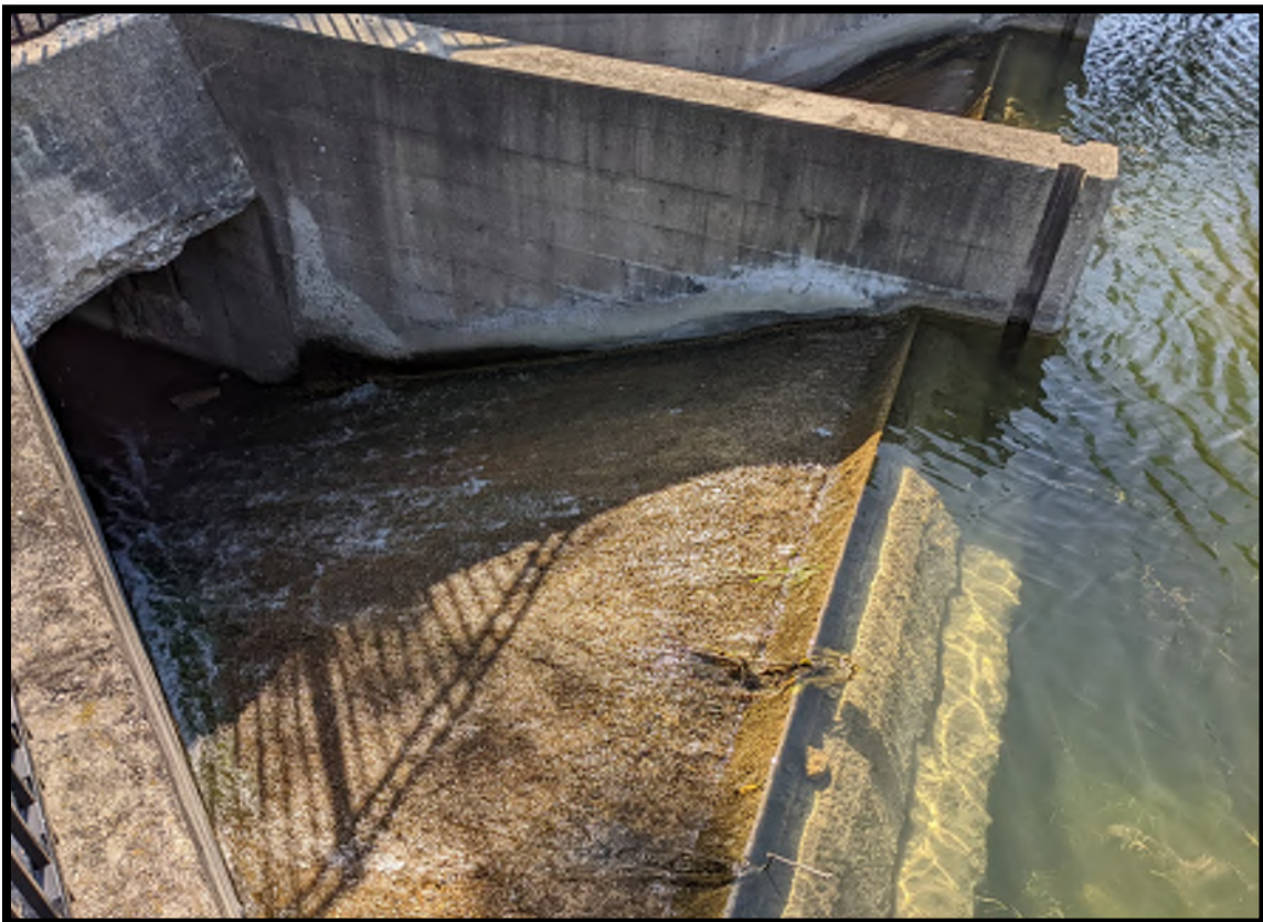
View of north chute with overflow into Honey Creek 0021006162202.jpg
