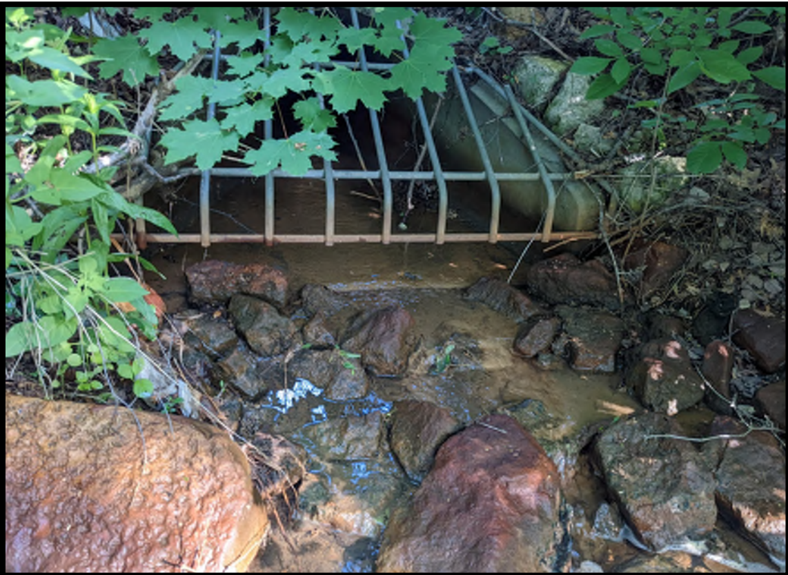
Outfall sewer pipe from Sterlingworth Bay 0021006162212.jpg
