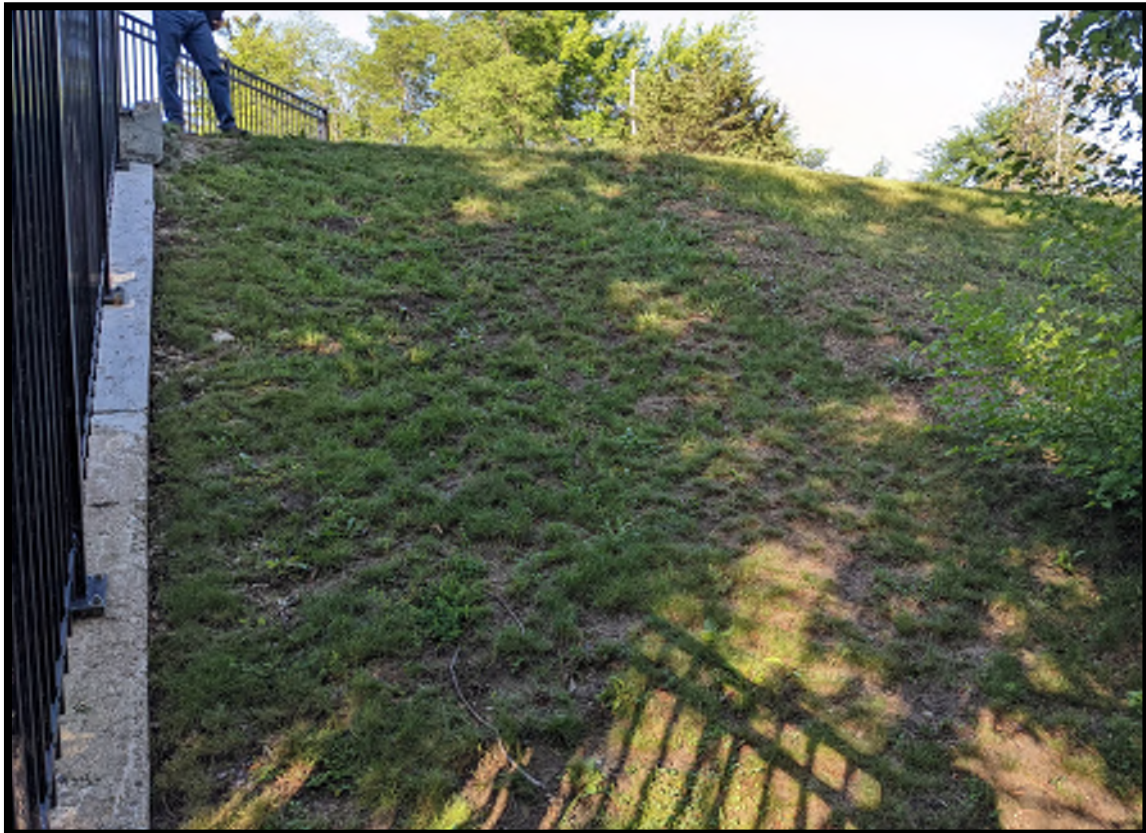
West (right) embankment looking upstream 0021006162204.jpg
