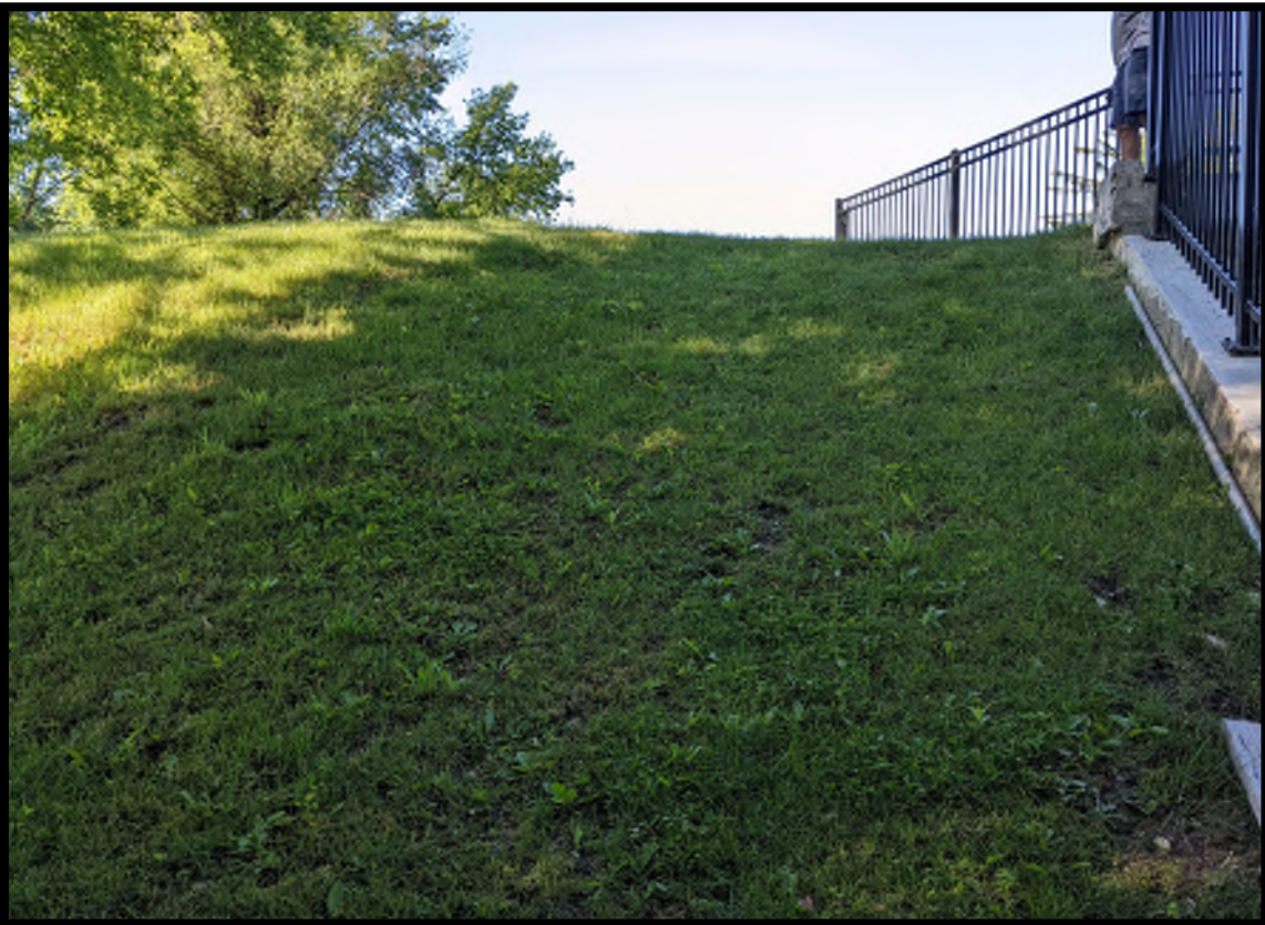
East (left) embankment looking upstream 0021006162206.jpg
