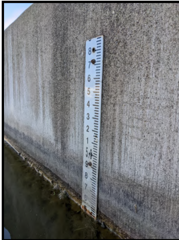
Gauge on upstream culvert headwall 0021006162210.jpg
