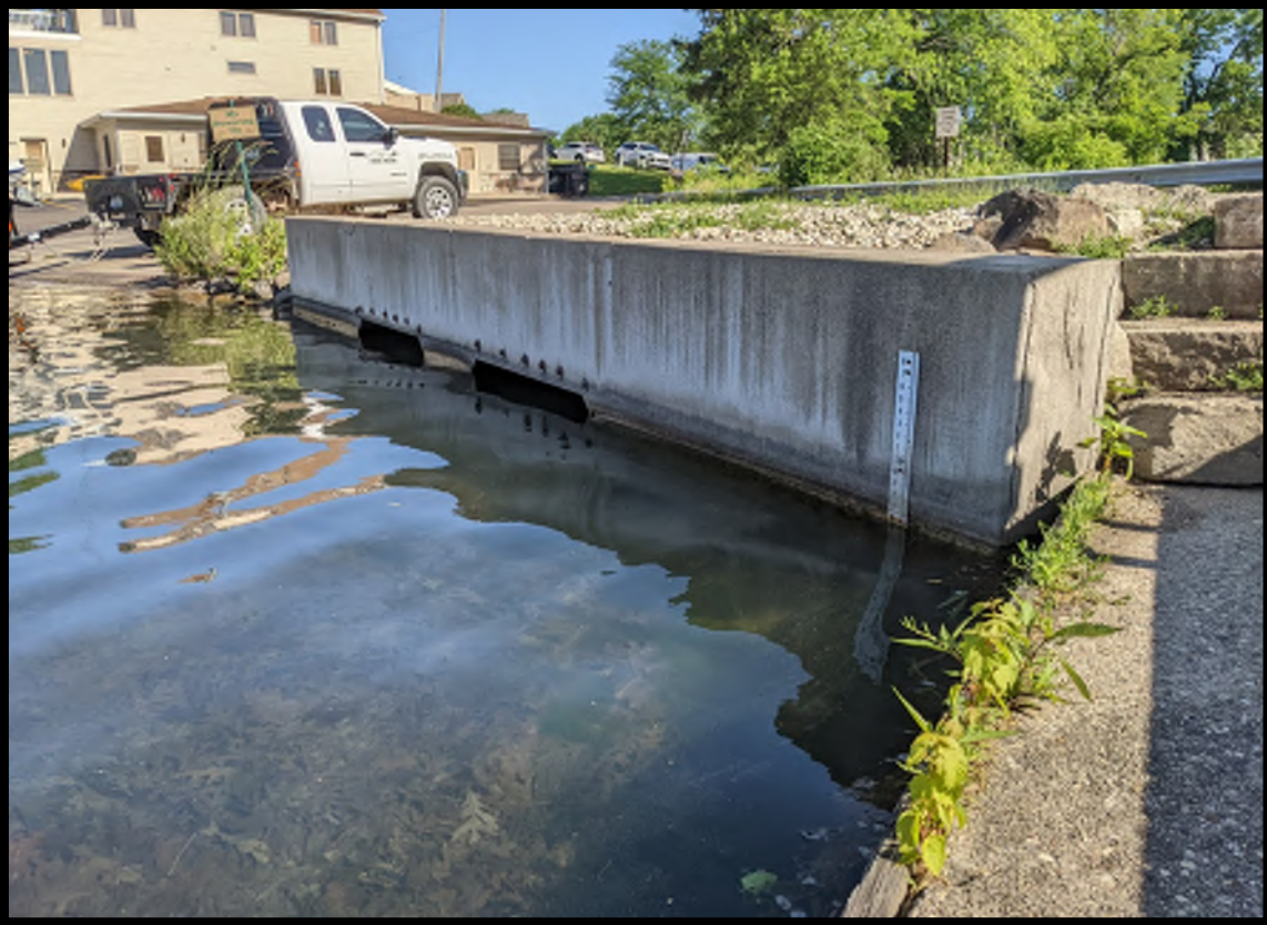
Upstream headwall and culverts 0021006162209.jpg
