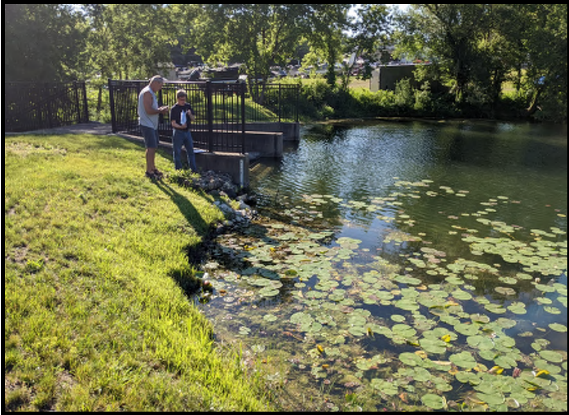
Upstream view of primary spillway from north bank 0021006162201.jpg
