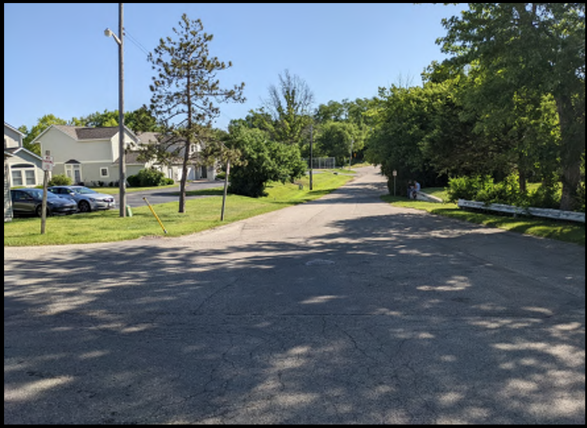
Roadway portion of Sterlingworth Bay embankment 0021006162213.jpg
