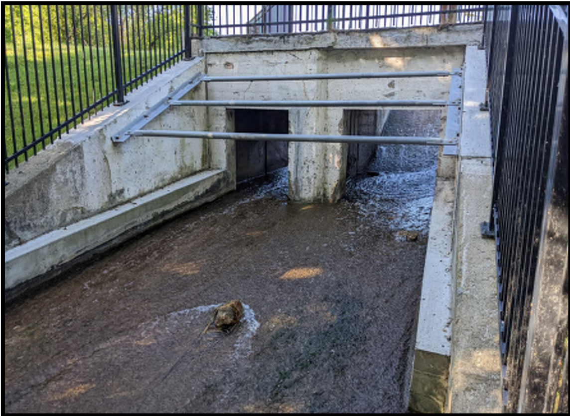
Downstream view of dam (former location of powerhouse) 0021006162208.jpg
