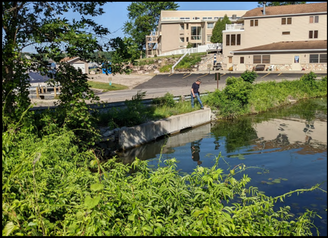
Downstream headwall and culverts 0021006162211.jpg
