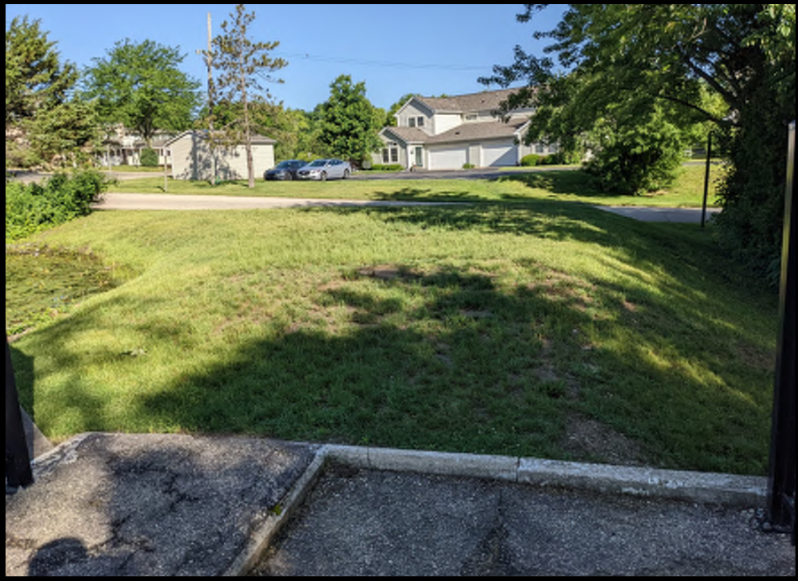
West embankment looking northwest 0021006162205.jpg
