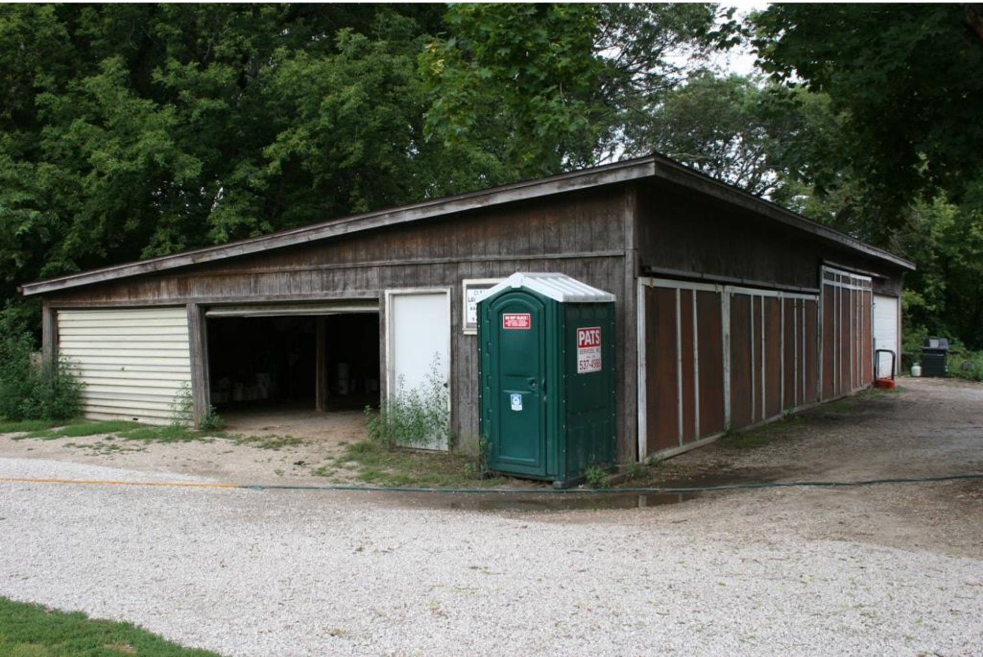
2006 Built Maintenance Building
